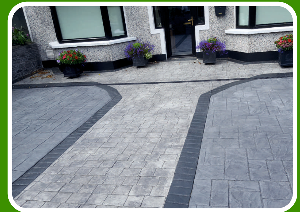
Entrance Footpath is London Cobble in a Silver Grey with a Charcoal R/A. Pattern on Either Side is Ashlar Stone in Platinum with Classic Grey R/A
