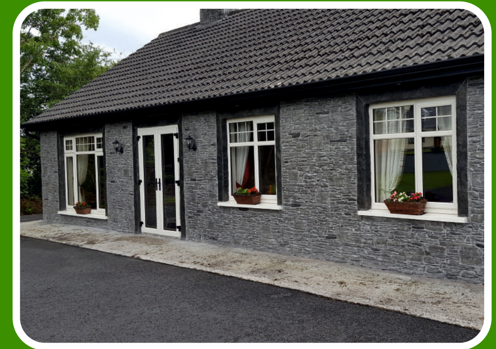
Bungalow with Imprinted Walls in Dry Mounted Stack Pattern
